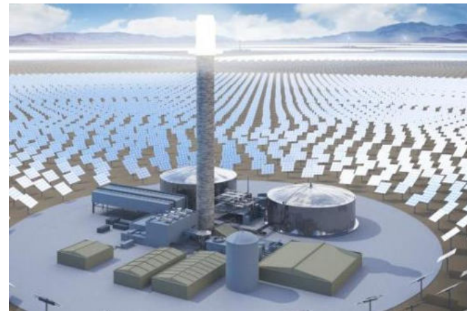
Crescent Dunes Solar Energy Project
