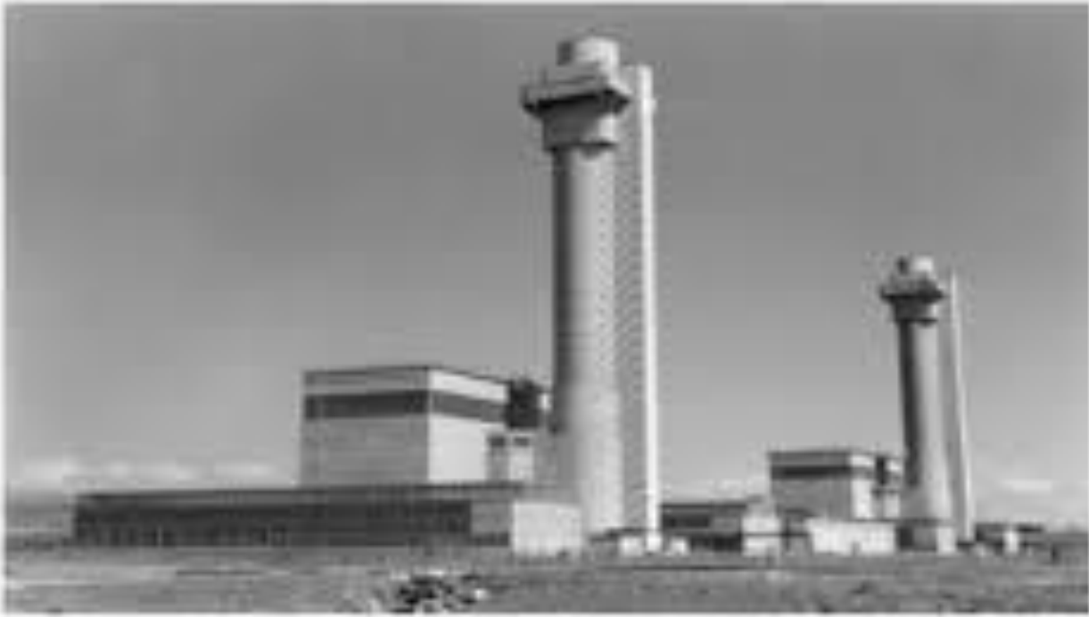
Windscale Air Cooled Piles
